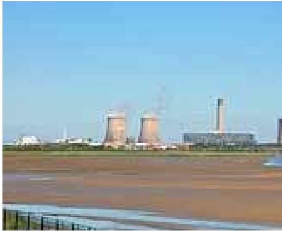
Coal fired power station
