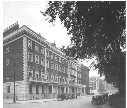
Figure 3. 1950s view of buildings surrounding Gordon Square. (Source: National Monuments Record)
